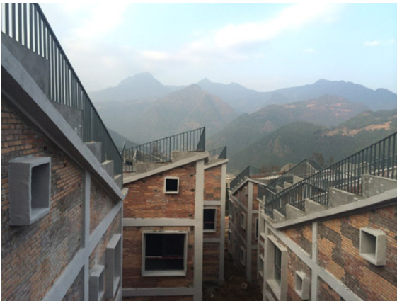
Rural Urban Framework’s Jintai Village homes were developed with stepped roofs to be planted with gardens
