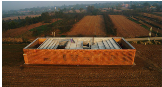
Rural Urban Framework’s prototype village property in Shijia is wrapped in a brick display, which provides ventilation even though safeguarding the interior mud walls
